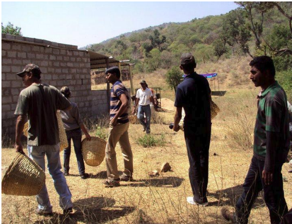
Image 2.6 A new building at Dabaguli
